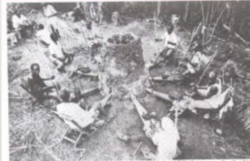
In the center, ceramic blowpipes—called tayere —are placed at the base of the furnace over the pit, which has been filled with charred swamp reeds and other charcoal. These blowpipes will serve as a conduit for the air forced into the furnace and protect the air as it passes through them. At far right opposite, the furnace is constructed of large chunks of refractory slag consumed by termite mud. (Photo by Peter Schmidt)
