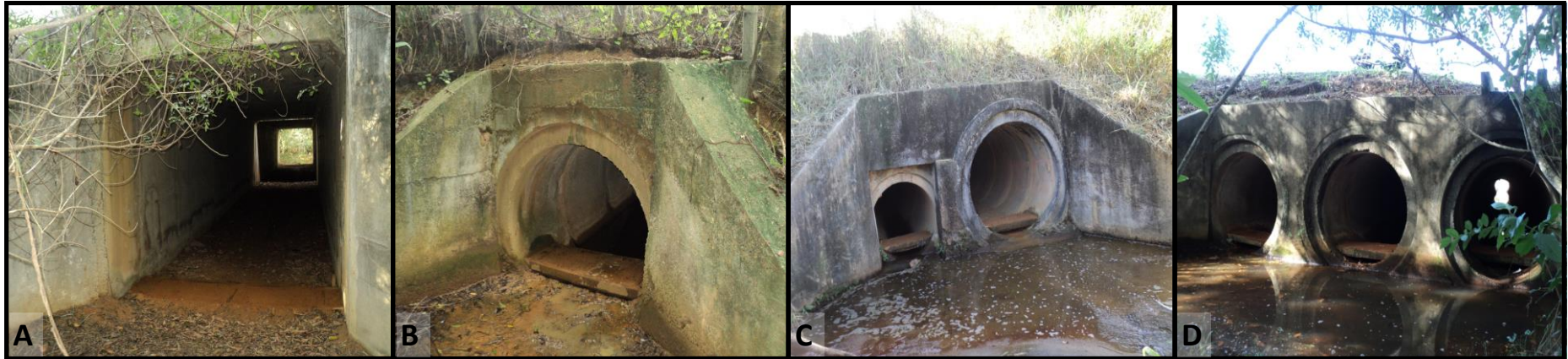
Figure S2. Representation of all types of underpasses installed on three mitigation clusters on Highway ES-060. (A) Single concrete box at km 45, (B) Single concrete culvert at km 45, (C) Double concrete culvert at km 59, (D) Triple concrete culvert at km 45.
